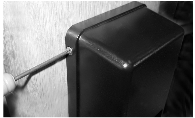
FIG. C: SECURE TOP OF "INSIDE HOUSING"
