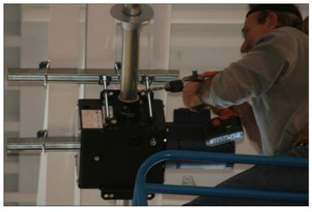
Figure 18: Securing the Drive Pipe to the Winch
