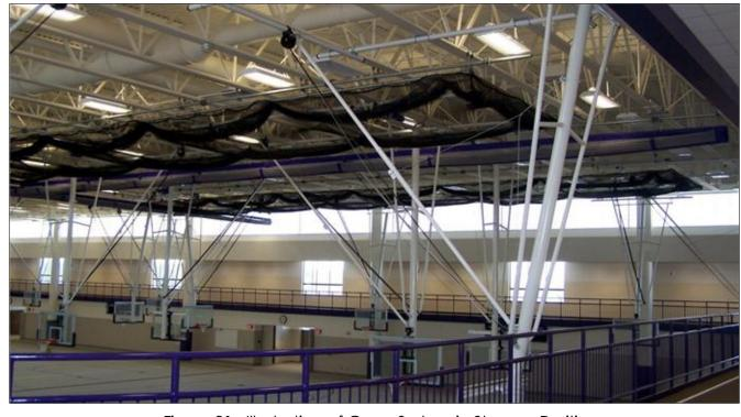
Figure 31: Illustration of Cage System in Storage Position
