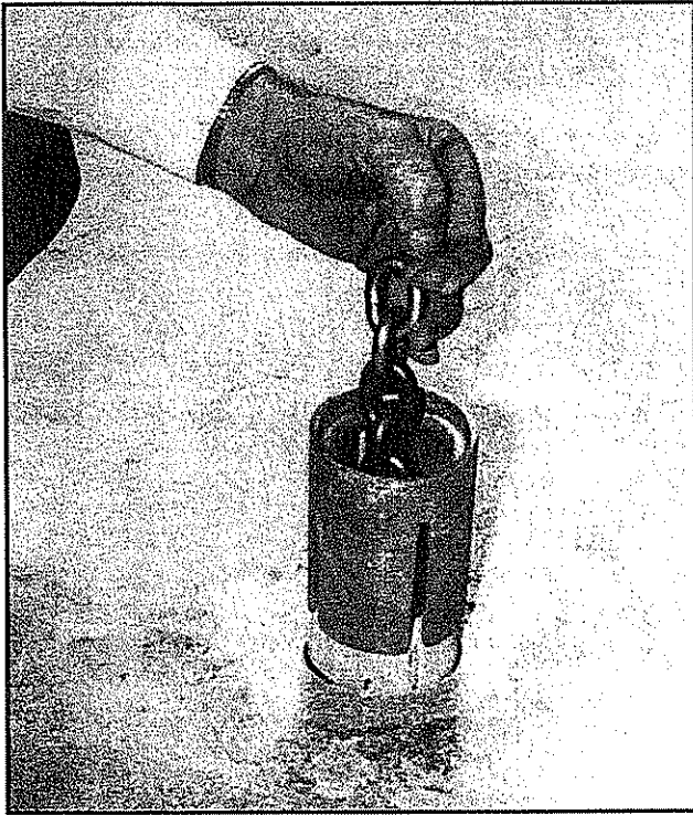
1. Insert assembled anchor into hole as shown. Use both hands if necessary.
