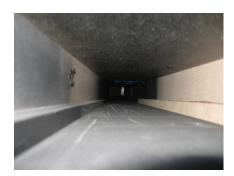
Ball return liners should be firmly glued in place with NO bubbles or wrinkles.
