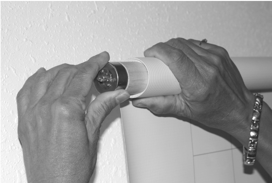
Use two hands to roll the screen back up onto the roller to tighten spring action.
