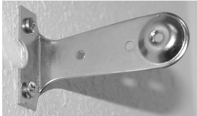
Right hand bracket, properly mounted
