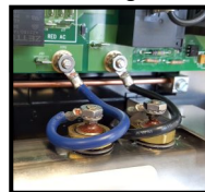
Replacement HQ heater wire kit installed
