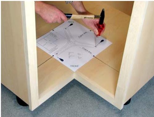
3. Mark the drilling holes
