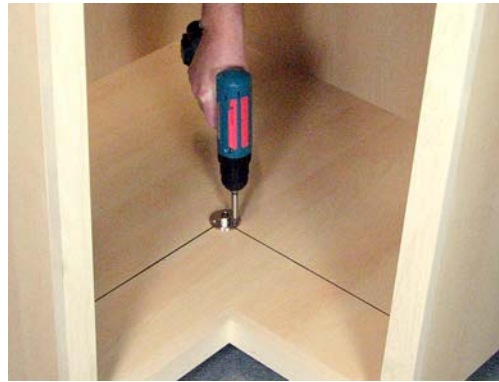
4. Mount the bottom bearing
