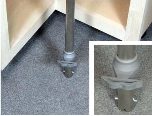
1. Mount bottom shelf support and bolt
