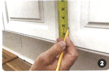
2 Measure from bottom of door to mark
