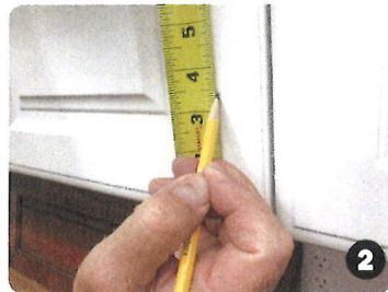
2 Measure from bottom of door to mark
