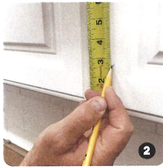
2 Measure from bottom of door to mark
