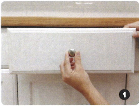
1 Place hardware (measure as needed) to find position you like; mark hole location (We are centering on width and height)
