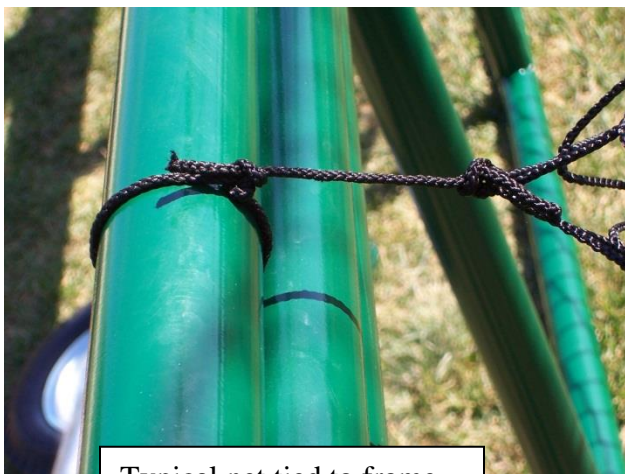
Typical net tied to frame.
