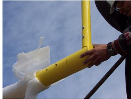
Once complete, repeat on the other side. After both goalposts are installed use yellow rustoluem to paint all of the bolt heads and all of the nuts. This will give the fasteners an extra layer of protection and it will give the goalpost a finished look, and also touch up any scratches.
