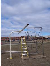
Insert crossbar into gooseneck. Set crossbar depth so the front edge of the crossbar is inline with the inside edge (field side) of the end line. Once the crossbar is level, mark (by using a center punch) and drill the holes through the gooseneck. Start with a 3/16" bit, then a 3/8" bit and finally a  $\frac{1}{2}$ " bit.
