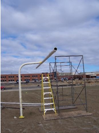
Insert crossbar into gooseneck. Set crossbar depth so the front edge of the crossbar is in line with the inside edge (field side) of the end line. Once the crossbar is level, mark (by using a center punch) and drill the holes through the gooseneck. Start with a 3/16" bit, then a 3/8" bit and finally a 1/2" bit.
