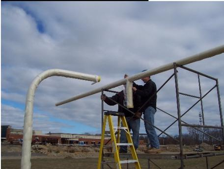
Use 10' scaffolding and a ladder, have two people on the scaffolding to lift and move the crossbar. Now with a third person on the ladder guide the insert into the gooseneck.
