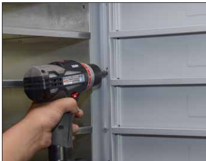
Figure 16– Secure units together using connector machine screws
