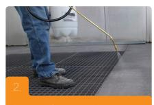
Apply a uniform coat with a pump sprayer.
