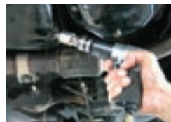
DRILLING DRAIN HOLE
