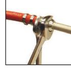
**Tighten compression** union onto aluminum line.
