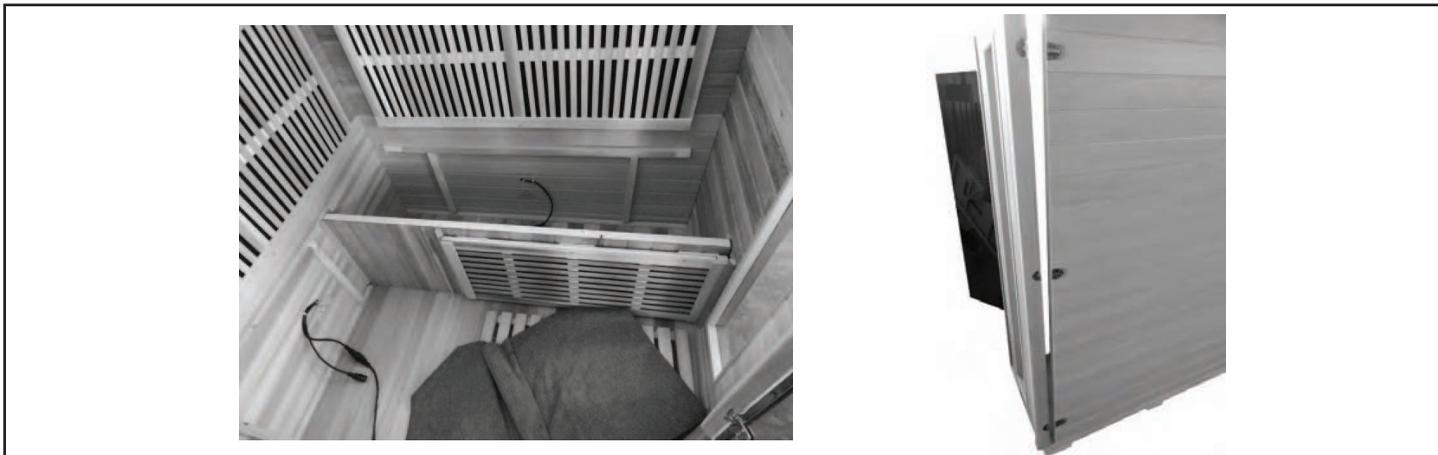
8. Slide the SHORT BENCH HEATER PANEL into place between the LONG BENCH HEATER PANEL and LEFT PANEL. Connect the heater plug. *Note: Make sure the FLOOR HEATER cable is placed through the groove in the bottom of the SHORT BENCH HEATER PANEL.*
