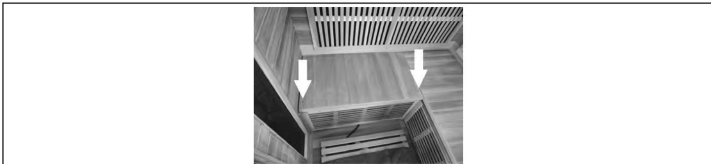
11. Lift the ROOF above the sauna, feeding the control panel and heater cables through the corresponding holes. Feed the cables for the AM/FM CD PLAYER through the hole in the bottom of the ROOF. Secure the ROOF to the sauna with 1-1/8" SCREWS. Connect the control panel and heater plugs.
