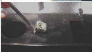
10. Fit M8 cage nuts for stone tray in four positions to inside face of lower pan.
