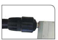
Slide WPS-7 over the JMA 1-5/8" DM connector, making sure to overlap the dedicated 1-5/8" port seal.
