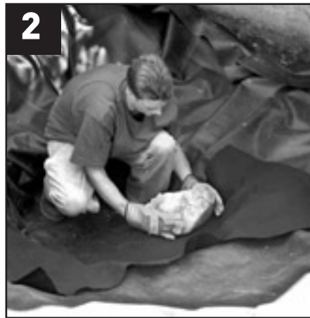
2 Place rockwork to form a border along the edge of the bog shelf.
