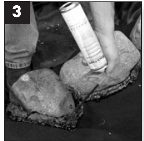
3 Use a bead of black foam to secure and seal the base of the rockwork.
