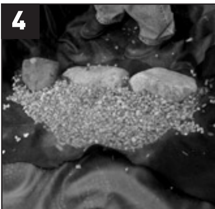
4 Fill behind rockwork with \frac{3}{4} " - 1 \frac{1}{2} " stones.
