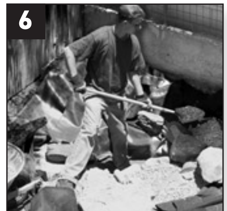
6 Add foam and more stones Note: The bottom of the pond should be kept smooth for easy waste removal.
