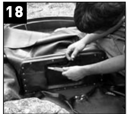
18 After the faceplate is properly tightened use a knife to trim the liner inside the mouth of the Skimmerfilter™.
