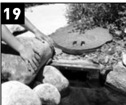
19 Hide the Skimmerfilter™ from view by extending the coping shelf rockwork to both sides of the Skimmerfilter™ opening.
