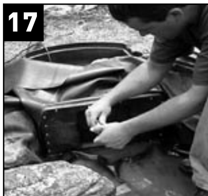
17 Use a #3 phillips head screwdriver to install screws halfway into all four corners. Install the remaining screws halfway. Tighten top, bottom and sides alternately by hand until screw heads are flush to create a watertight seal.
