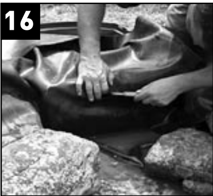
16 A) Make a 3" wide incision through the centered liner \frac{3}{4} " below the top of the Skimmerfilter™ opening. B) Slide the faceplate over the locator pins to align the screw holes.
