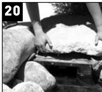
20 Place a flat rock over the Skimmerfilter™ neck to camouflage.
