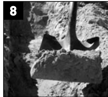
8 Use backfill dirt to hide the Kink Free Hose.™
