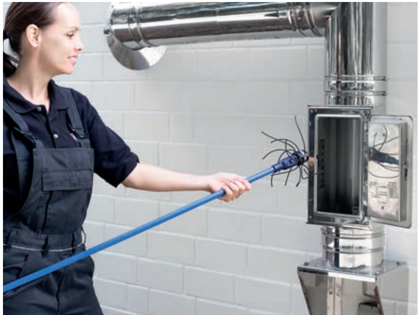
Stainless steel chimneys can be cleaned gently with the nylon wires.
